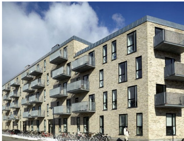
EXAMPLE OF BALUSTARDE TO UPPER FLOORS
