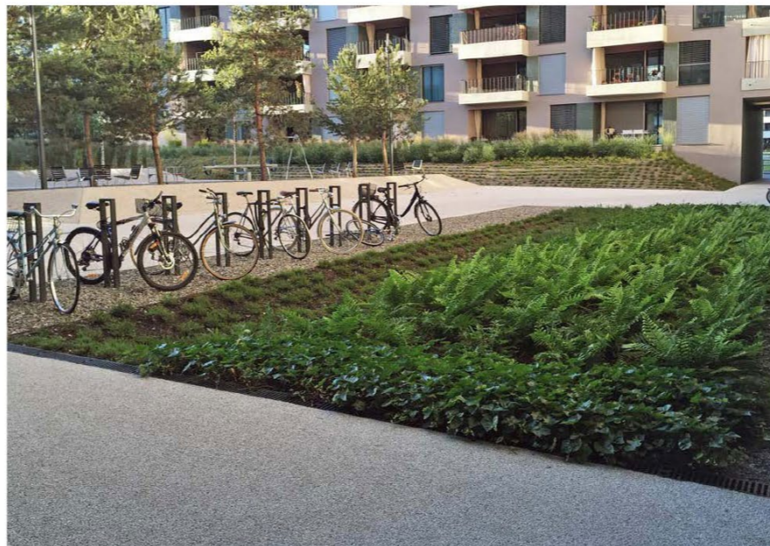
Residential courtyard - in situ concrete paved circulation with firm gravel to bicycle stands
