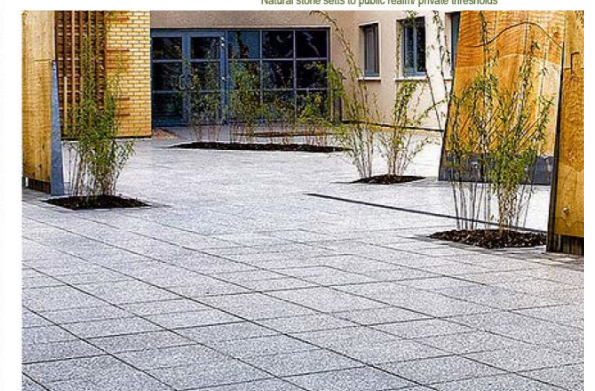
Pre-cast concrete pavers to residential terraces and podium garden
