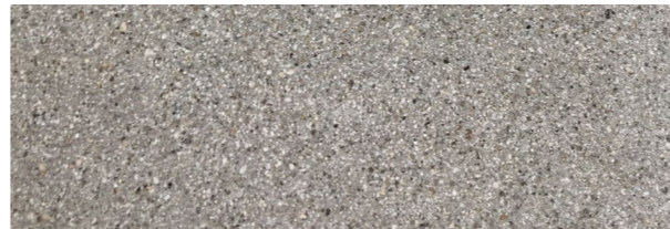
Reconstituted stone cladding to lower levels
